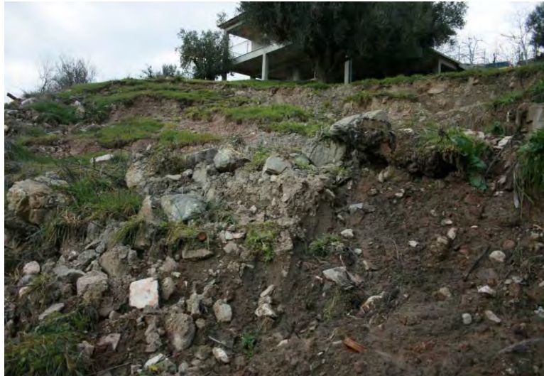
Figure 3. Photo of the landslide taken from the southeast. The head of the landslide is in front of two olive trees about two meters from the house basement.
