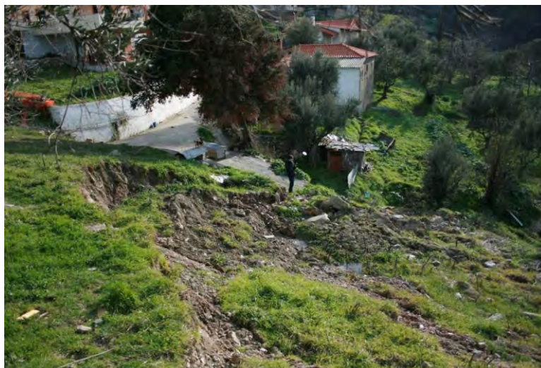
Figure 4 - Photo of the landslide taken from the northwest. Part of the small village road is collapsed.
