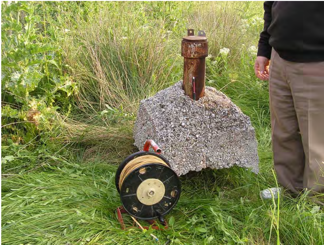
Figure 3 - Well-casing protrusion, of about 20cm. The current well is located next to the G2 main well (Figure 6).
