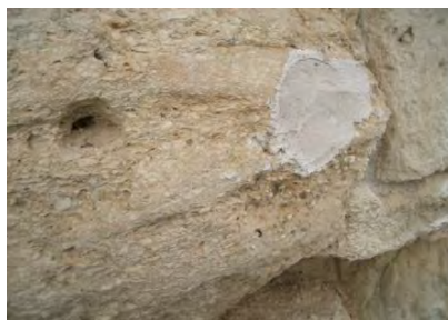
Figure 3 - Sampling position of a building stone from the internal wall of Koule Castle. The drill hole was covered with a non compatible mortar.
