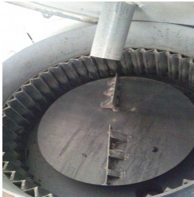
Figure 3 - Inside view of the centrifugal crusher.
