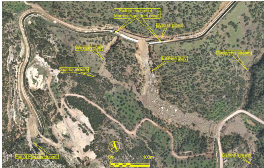
Figure 1 - Aerial view of the slide area.
