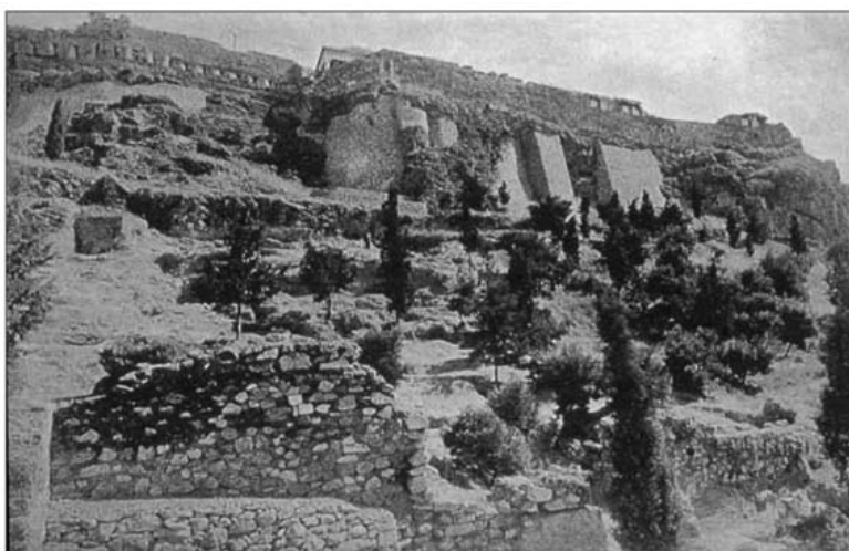
Fig. 1: The North bank of the Acropolis of Athens, (after Broneer, 1939).
