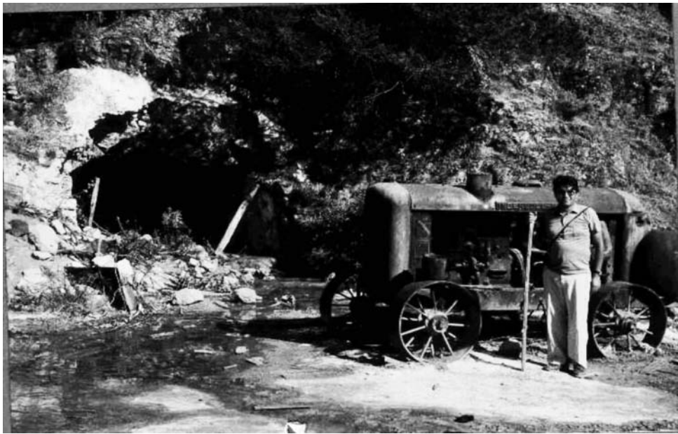
Fig. 3: Acid drainage related to pyrite oxidation (from Hermioni mining area Greece).
