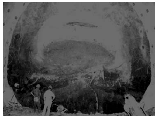
Fig. 7: Old collapsed tunnel during re-excavation.
