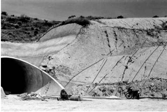
Photo 1: Southern portal of tunnel SB (left branch). The two units (Upper and Lower ones) are distinguished, due to color and structure. Their continuity is interrupted by faults that considerably change dipping.
