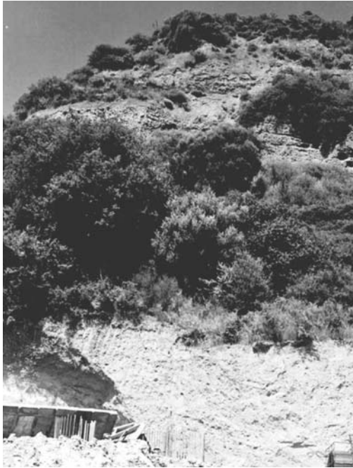
Photo 3: Exit of SG tunnel. Stratigraphic column of the Upper Geotechnical Unit at the base, overlaid by conglomerates with distinct bedding (Unit of Argillaceous marls with coarse-grained material).
