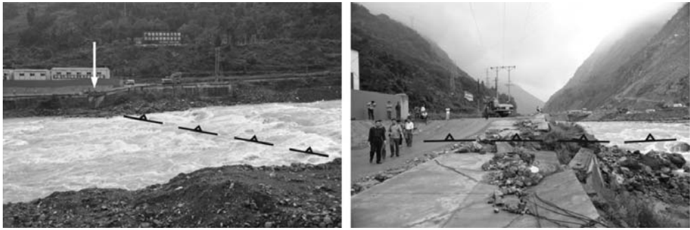
Fig 5: Views of the Yingxiu-Beinchuan seismic fault at the outskirts of Yingxiu town.
