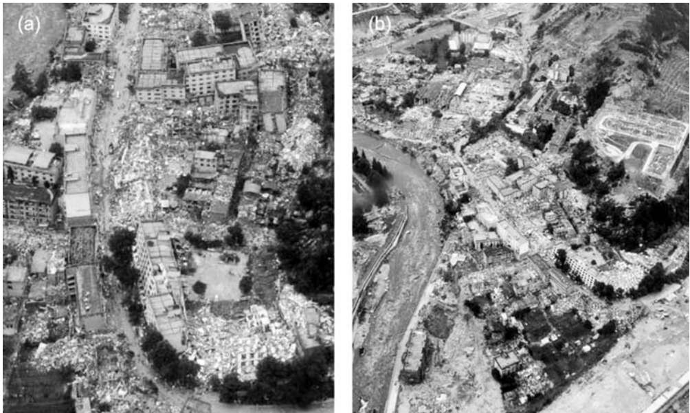
Fig. 4: Oblique aerial view of residential constructions in the Wenchuan and Beinchuan towns that suffered total destruction. These towns were founded on river terraces in the mountainous region. Large scale landslides on the surrounding slopes contributed to the destruction of the residential constructions (Xinhua News Agency China 2008, Reuters 2008).
