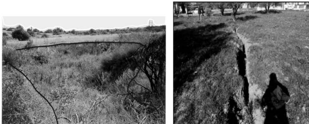
Fig. 5: a) left – An old sinkhole in a riverbed , b) right – Linear ground cracks.
