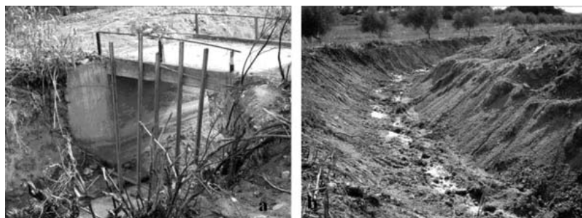
Fig. 8: Debris Rack (metallic fence) (a), widening and clearance of river network (b).
