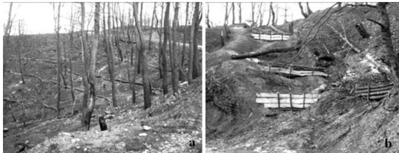
Fig. 7: Log or brunch barriers (a) and small wooden dams (b) for soil erosion protection.
