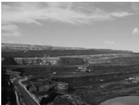
Fig. 5a: PPC Lignite mine for el. power generation.
