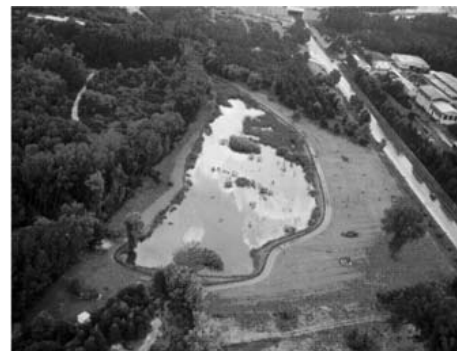
Fig. 5b: Environmental rehabilitation of open pit
