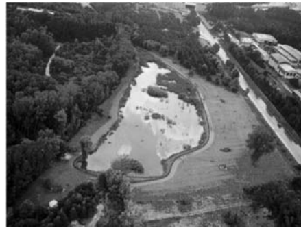
Fig. 5b: Environmental rehabilitation of open pit
