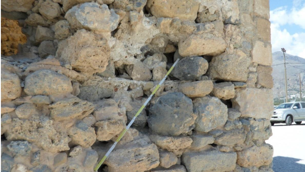
Figure 3 - Various rock types in the masonry walls.
