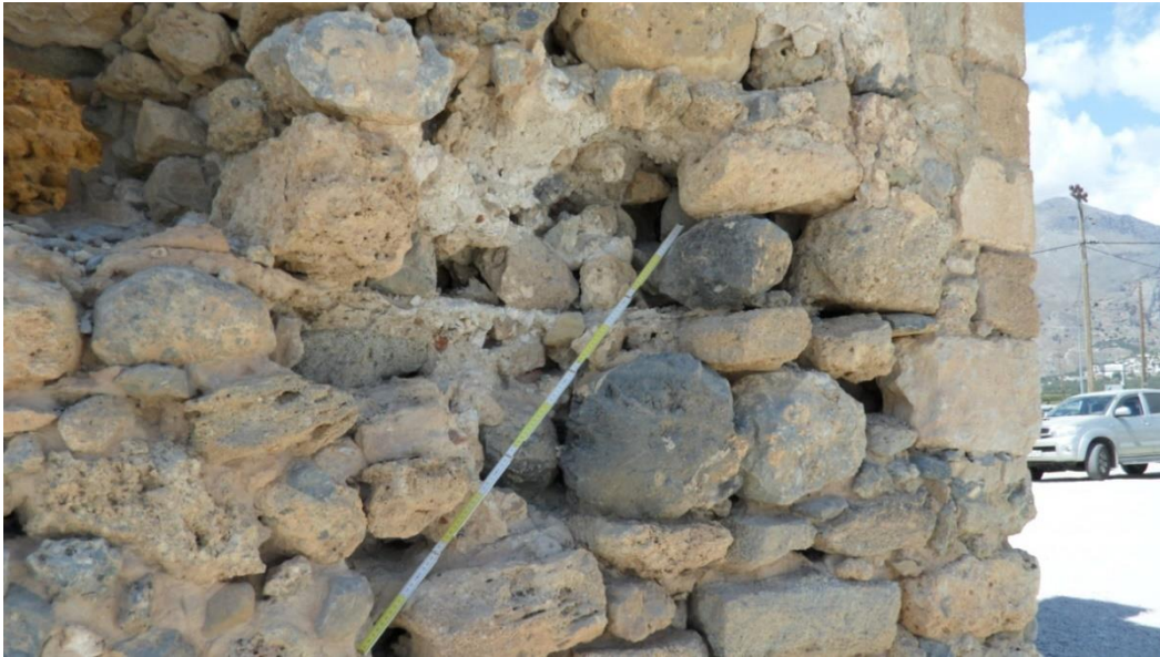
Figure 3 - Various rock types in the masonry walls.
