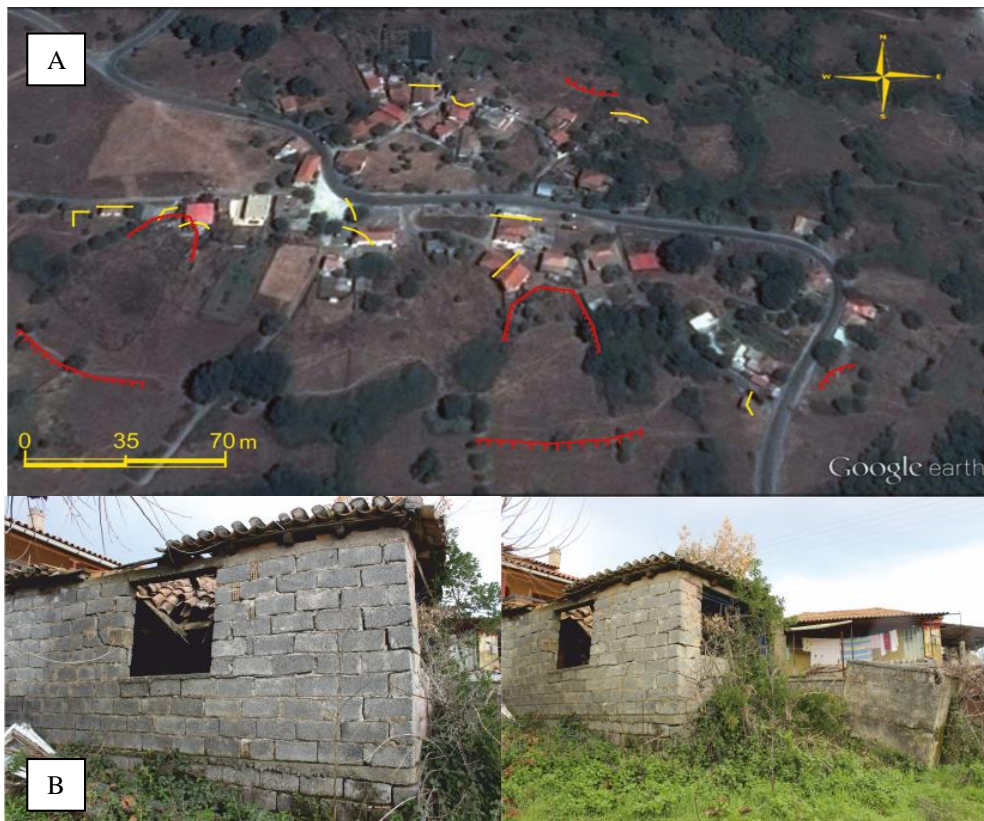
Figure 2 - A) The distribution of the failures. Slope failures are marked red, while failures in structures are marked yellow. B) Damaged buildings across the village.
