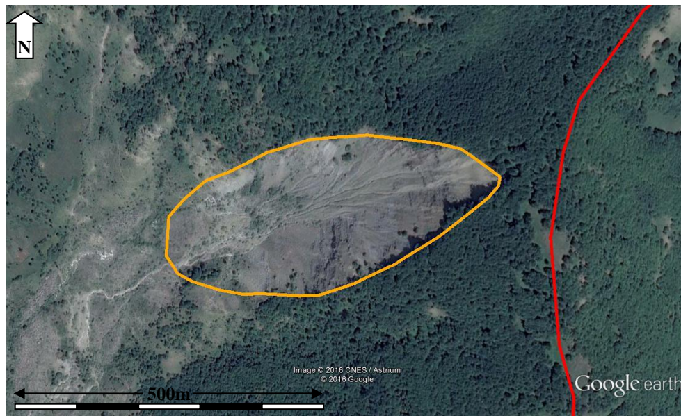
Figure 9 - Overview of a geohazard area (orange line) in close proximity with a proposed pipeline RoW (red line). In such cases, avoidance by rerouting is the preferred option. When the landslide hazard is not avoided, it must be feasibly constructed, with reasonable low risk or reasonable engineering remedial measures.
