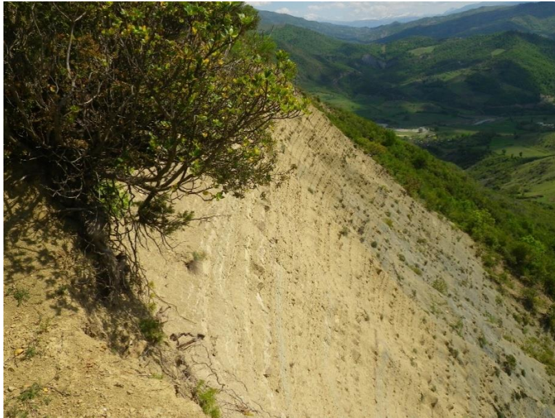
Figure 3 - Very steep landslide back scar extending to the ridge crest, with potential for further upslope retrogression.
