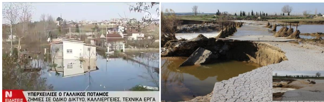
Figure 8 - Indicative damages caused by floods in Gallikos river basin.
