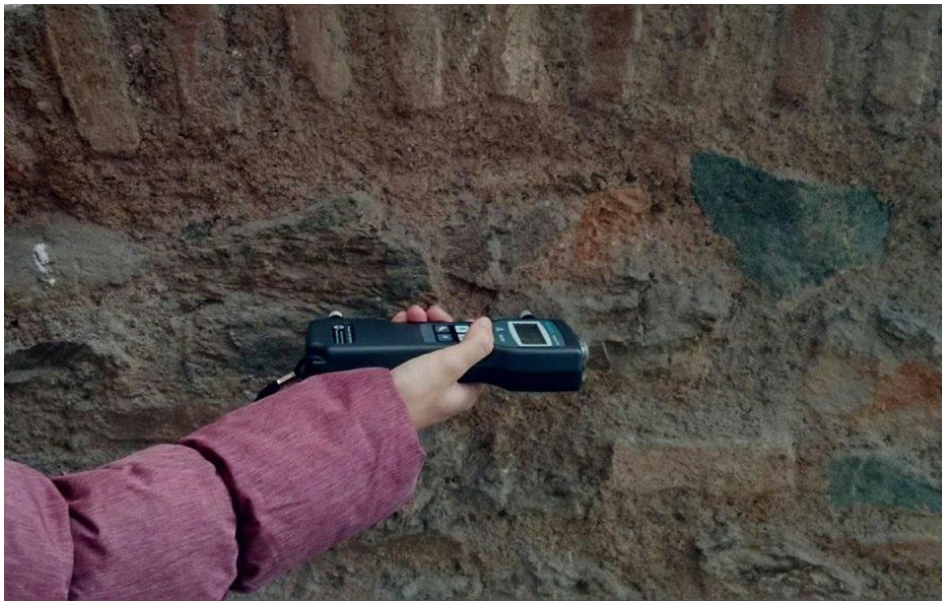
Figure 5 - The use of SURFER device on the monument.
