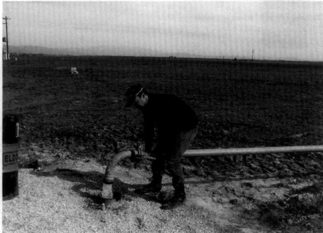
Figure 4 –Water recharge injection system
