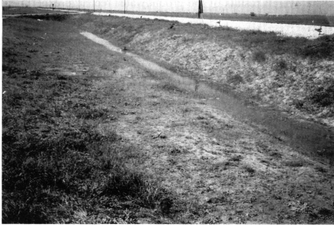
Figure 5 –Water recharge system through trench
