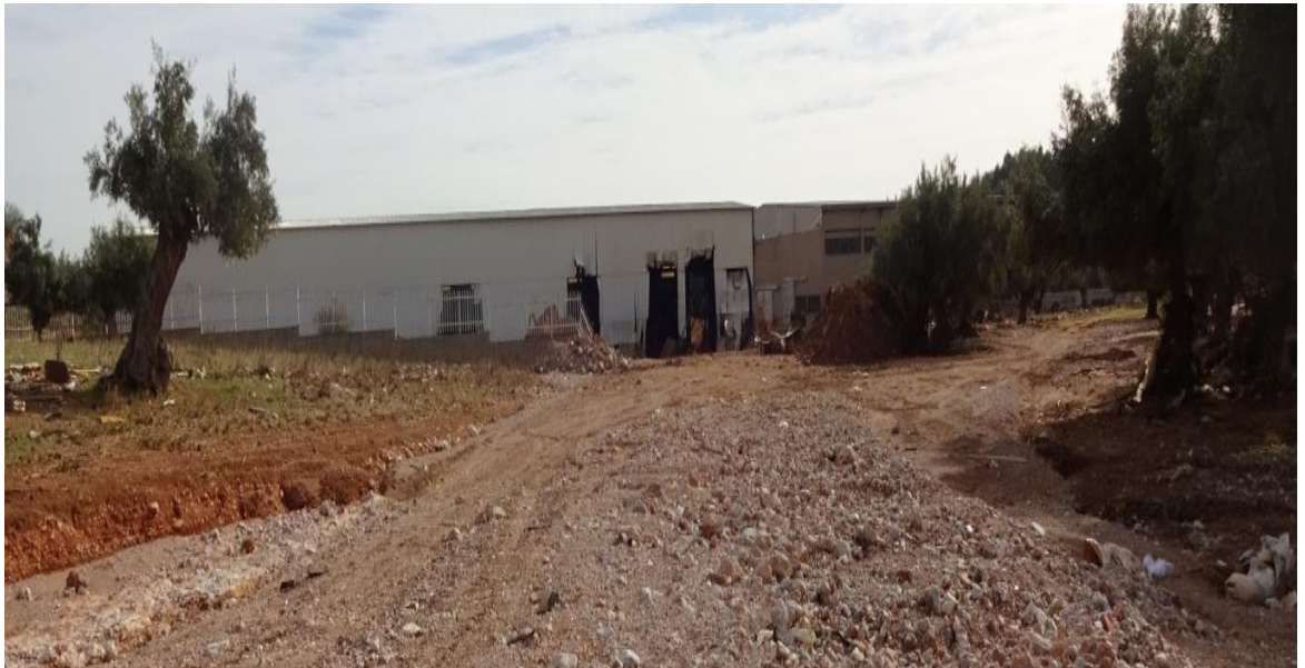
Fig. 5: Photograph of the Soures streambed which shows the existence of a massive building across the flow of the stream.
