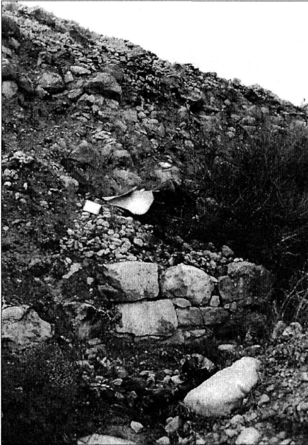
Photo 1. View of the Mycenaean dam with remnants of the eastern retaining Cyclopean walls on the side of the active channel. The core fill is made of dirt and large limestone blocks.
