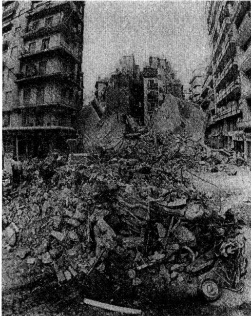
Figure 1. Building collapse in Thessaloniki after the 1978 earthquake
