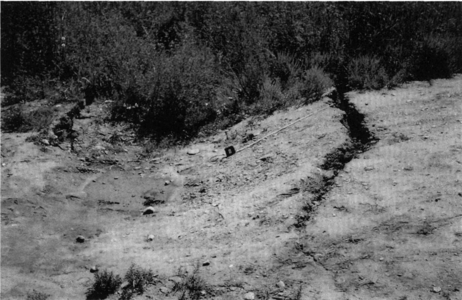
Figure 1 – The suffosion-subsidence processes above the underground sewer systems
