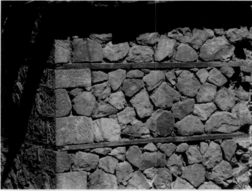
Figure 21 – Detail of house wall in Vrontero village
