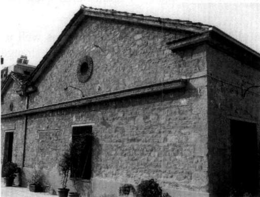
Figure 6 – Old cold store made of sandstone in Trikala town
