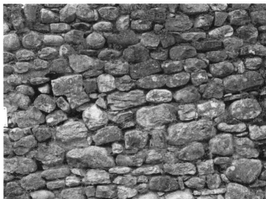
Figure 17 – Detail of the old bridge in Portaikos River
