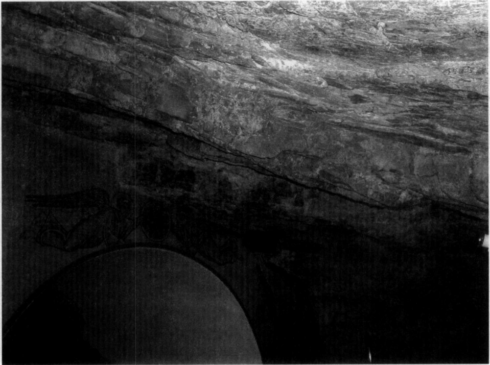
Figure 6 - Ceiling view of section A. Unsupported Section. This picture clearly presents a side view of the arc supporting section D, covered by hagiography
