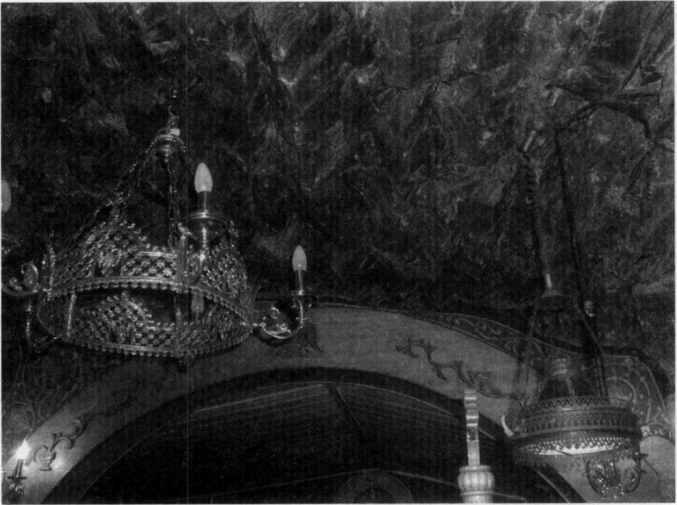
Figure 5 - Ceiling view of the Sanctuary and of section D. Sections supported by rigid arcs constructed by marble blocks and concrete. The Sanctuary is covered additionally by wood
