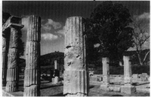
Figure 15 - Different degree of decay on column pieces
