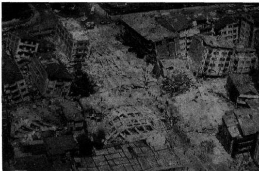
Fig. 3 Representative view of a portion of Adapazari that suffered total damage ( I_{EMS-98} = XII ) after the 17 th August earthquake.
