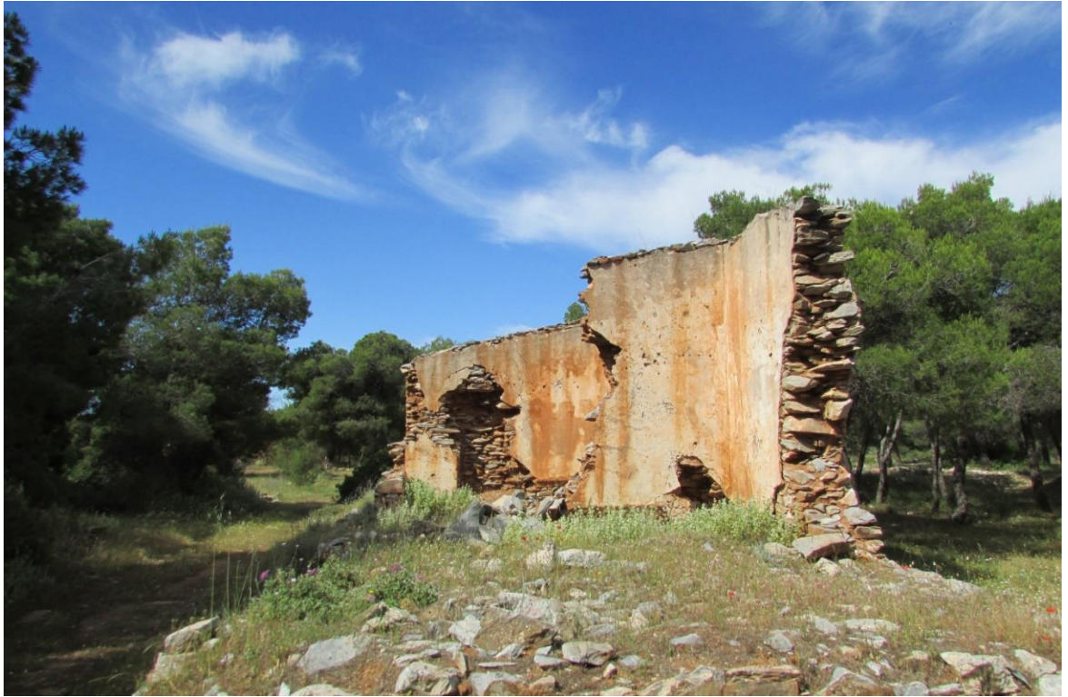
Fig. 5: Ruin of a mining installation at the Sounion National Park.
