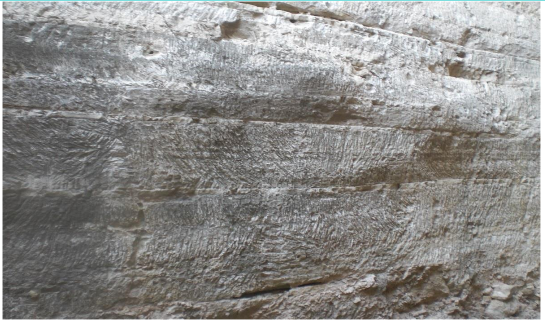
Fig. 6: Samos, Agiades hill. A quarrying pick with a sharp point used in smoothing out the sidewalls of a one-aisled underground quarry. Height of the outcrop approximately 2 m.
