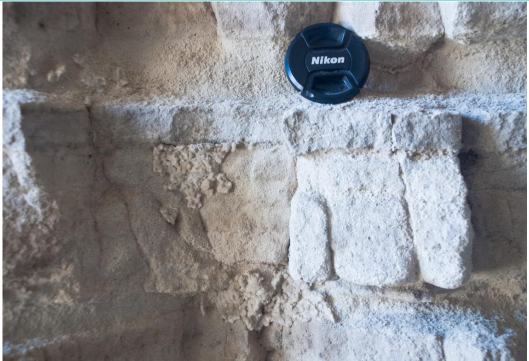
Fig. 4: Samos, Agiades hill. Niter ( \text{KNO}_3 ) still occurs as white fluffy material in fissures and joints of the beds in the lowermost row of galleries.
