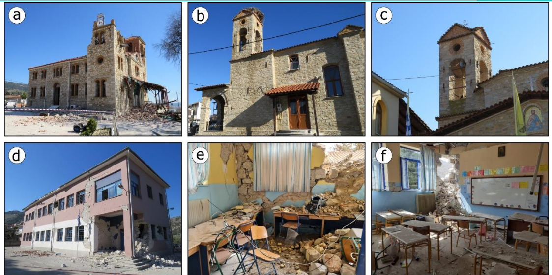
Fig. 8: (a) The Ayios Dimitrios church in Mesochori village, which has been founded on recent deposits, suffered damage to its walls and bell towers by the 3 March earthquake. The 4 March earthquake aggravated damage. (b, c) The Ayia Triada church in Vlachogianni village has been founded on alpine deposits and has been recently reinforced with steel ties in the bell tower and in the other parts of the construction. It remained intact by the early March earthquakes. (d, e, f) Damage to the old masonry elementary school of Damassi village. It suffered heavy structural damage including partial collapse of the walls.
