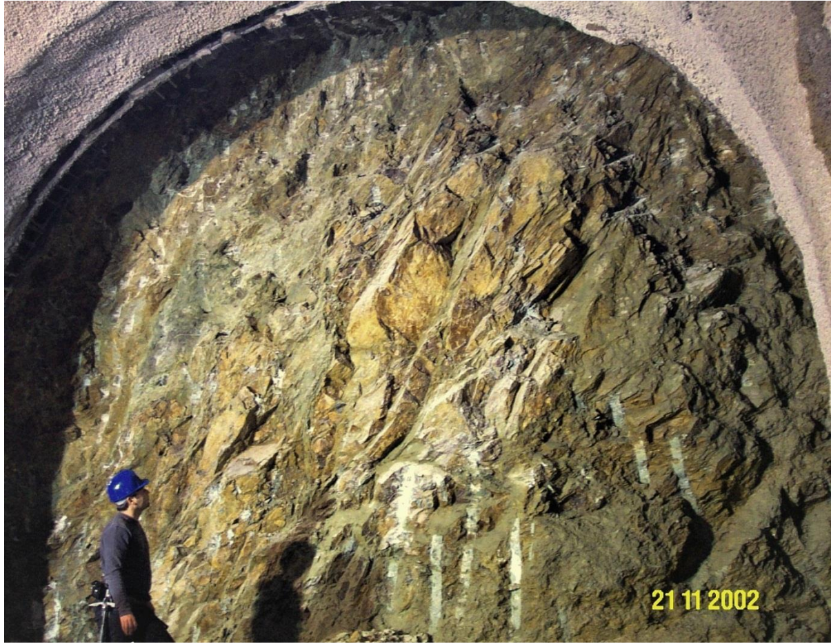
A.16 Olive green epidote-chlorite schist. Access tunnel (~ 6 m dia.) excavation face – Line 3, Thivon shaft, “Egaleo” - “Aghia Marina” interstation.
