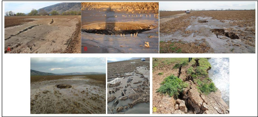
Fig. 12: Examples of sand flows, sand boils and lateral spreading in the liquefied area SE of Pineiada village.
