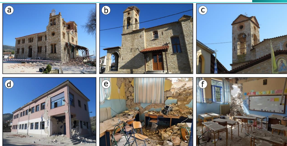
Fig. 8: (a) The Ayios Dimitrios church in Mesochori village, which has been founded on recent deposits, suffered damage to its walls and bell towers by the 3 March earthquake. The 4 March earthquake aggravated damage. (b, c) The Ayia Triada church in Vlachogianni village has been founded on alpine deposits and has been recently reinforced with steel ties in the bell tower and in the other parts of the construction. It remained intact by the early March earthquakes. (d, e, f) Damage to the old masonry elementary school of Damassi village. It suffered heavy structural damage including partial collapse of the walls.
