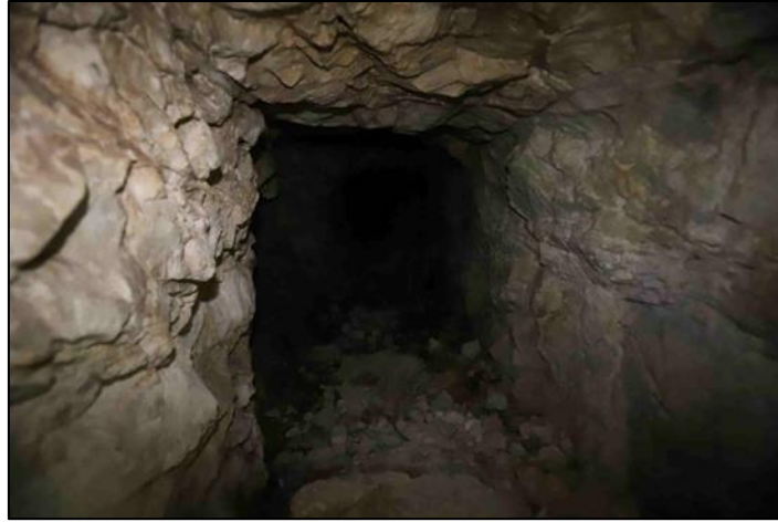
Fig. 10: Unfinished portico at Lisse Fort, constructed using conventional mining methods (Source: Personal file)
