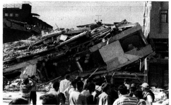
Fig. 4 Reinforced concrete frame structure that collapsed in Gölçök town (damage degree 5).
