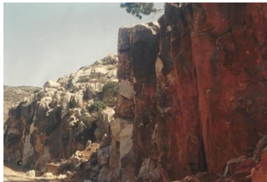
Figure 1. A road section near Chania (Greece) slightly tilting due to gravity.
