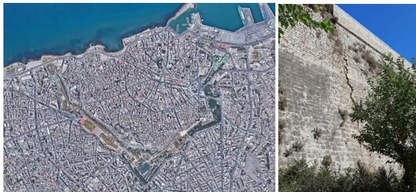
Figure 1. (a) A satellite image of the Heraklion City bastion fortification system (Google Earth) (b) The three (3) construction phases of the line-segment Bembo-Saint Francis can be easily distinguished. A vertical crack is also visible
