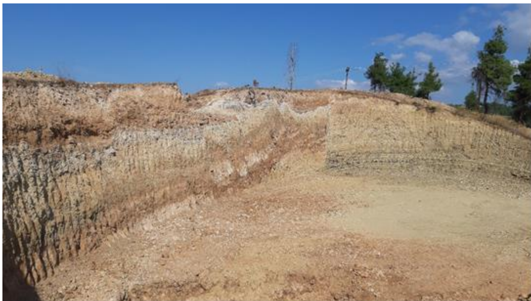
Figure 1. General image of the normal fault system revealed in the Water Tank D1 partial foundations excavations.
