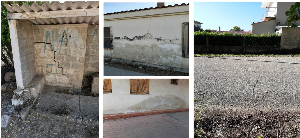
Figure 2. Indicative photos showing damages caused by land subsidence phenomena in Mavrogia (left photo), Aliartos (photo center-up), Agios Dimitrios (photo center-down), Alalkomenes (right photo)
