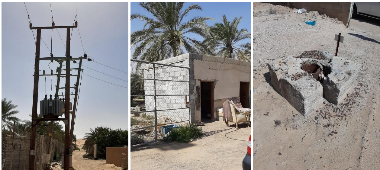
Figure 2: Deformations and the failures, proofs of the land subsidence. Dislocated Electrical pillars with their wires tensioned, differential settlements affecting buildings and protruding well casings, identified during the field observation
