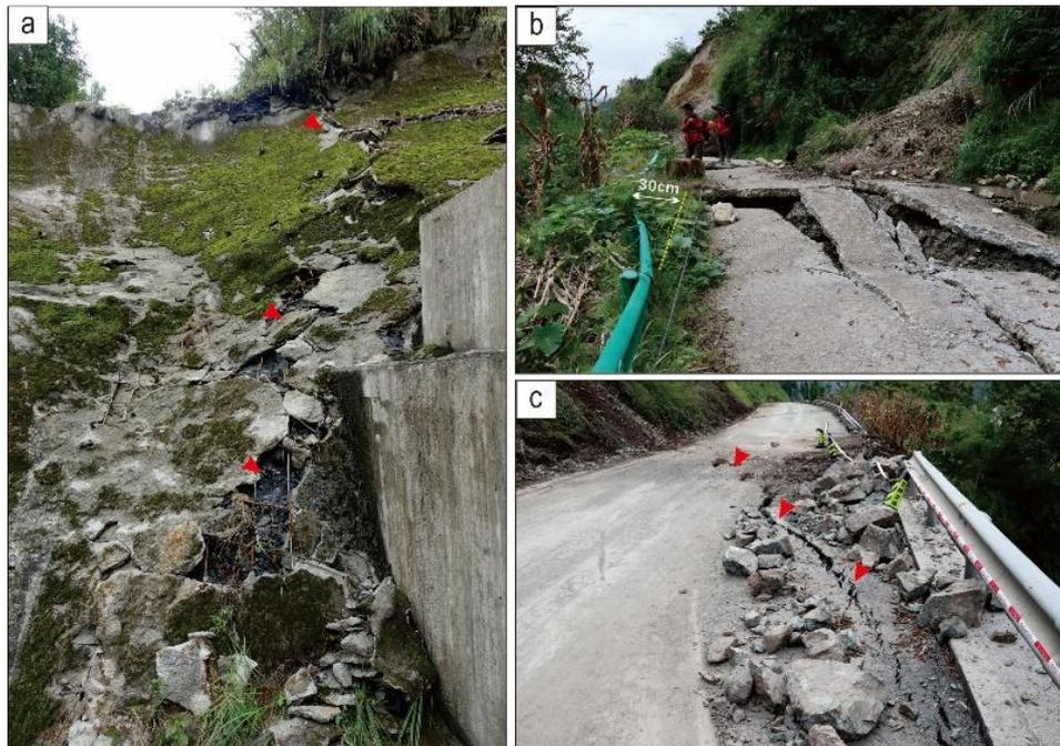
**Figure 3. Field photographs showing co-seismic surface ruptures from the Ertaizi to Aiguocun village.** (a) the Wandong village site, view to SE; (b) the Xingfucun village site, view to south; (c) the Aiguocun village site, view to south. See locations in Fig.2.
