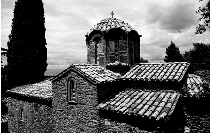
Fig. 7. A view of the katholikon of Asteriou monastery, with the characteristic so-called “Athenian type” dome, which imitates a Byzantine local architectural form.
