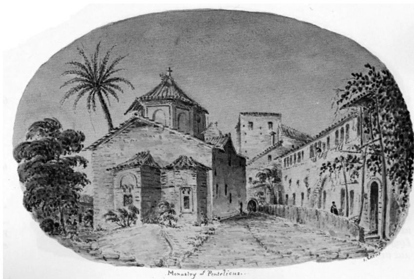
Fig. 6. A view of the katholikon and the north wing of the monastery of Penteli, by Skene, op. cit. , no. 61. Today these buildings have suffered extended alterations.
