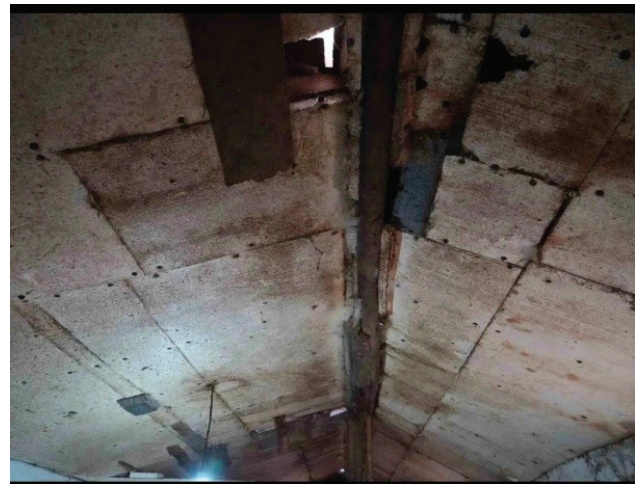
Figure 5. Styrofoam ceiling and ventilation of the sampled family barn in the İhsangazi District of Kastamonu Province (Photographed by Giray and Şimşek).
