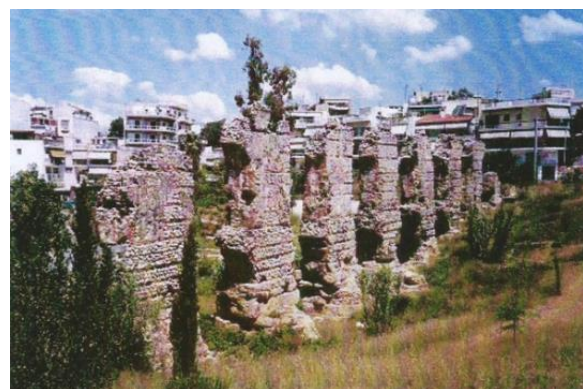
Figure 1. Photo of an overground part of Hadrian's aqueduct in Nea Filadelfeia (photo taken by H. Alexandri).
