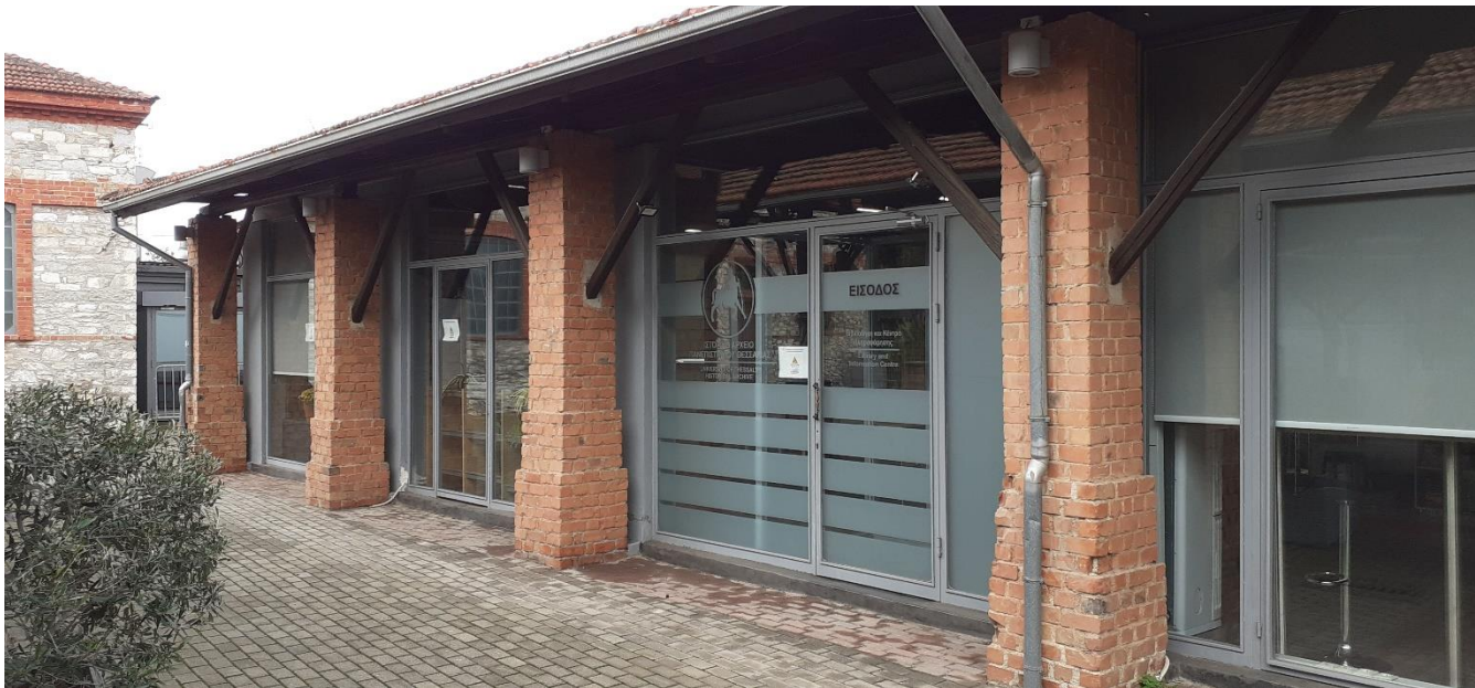
Fig. 1. The University of Thessaly Historical Archive building (Central Library branch) in the Tsalapata complex in Volos
