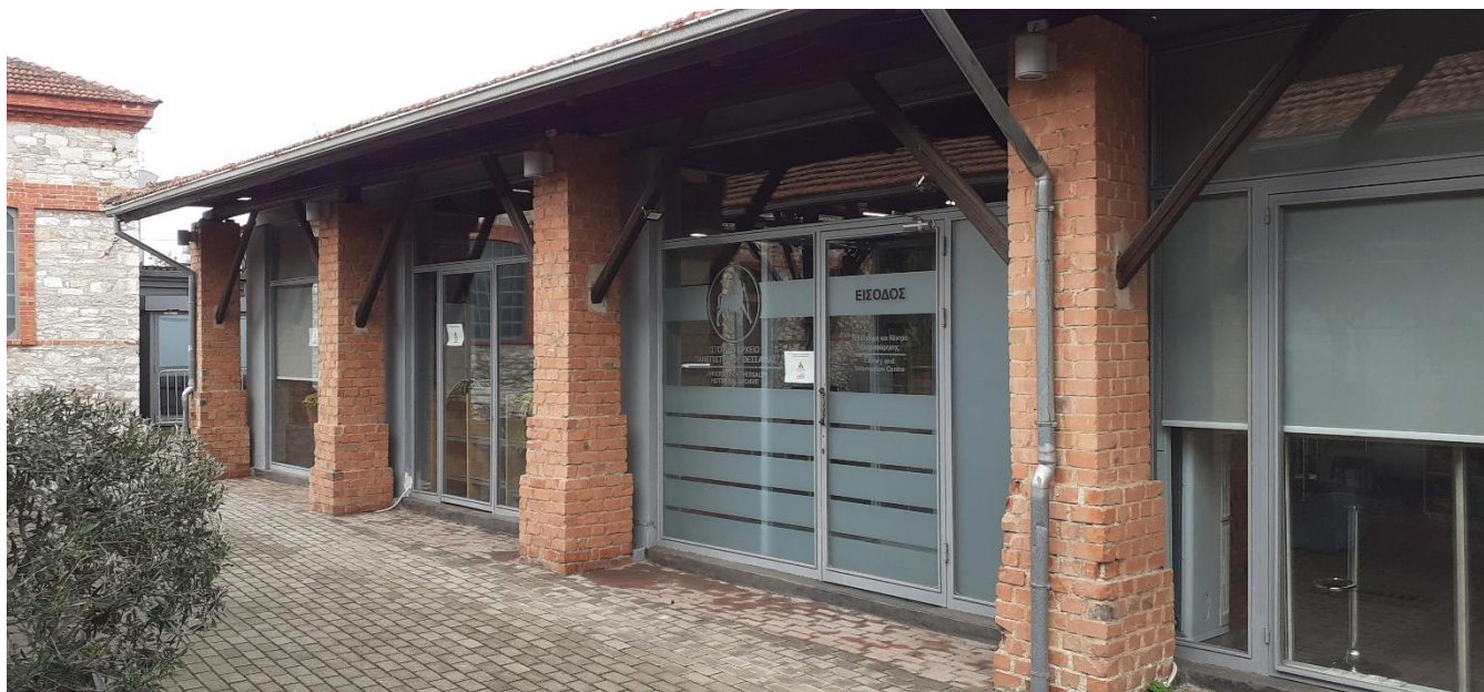
Fig. 1. The University of Thessaly Historical Archive building (Central Library branch) in the Tsalapata complex in Volos
