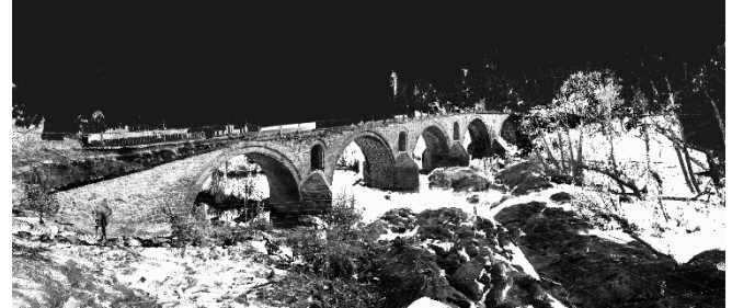
Fig. 3. Registered point cloud of the bridge of Spanos (image of the authors).
