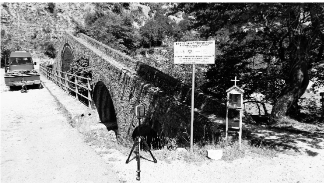
Fig. 2. Digitization of the bridge of Politsa using laser scanning (photo of the authors).
