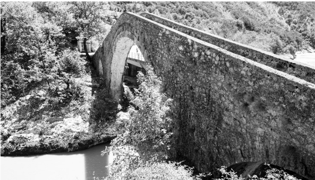
Fig. 11. The bridge of Politsa, current condition (photo of the authors).
