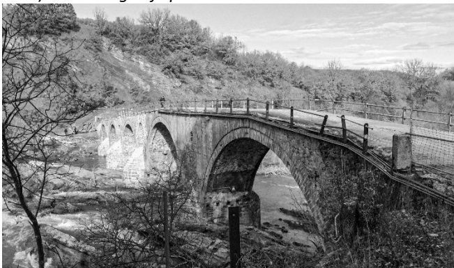
Fig. 7. The bridge of Spanos, current condition (photo of the authors).
