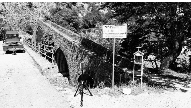
Fig. 2. Digitization of the bridge of Politsa using laser scanning (photo of the authors).
