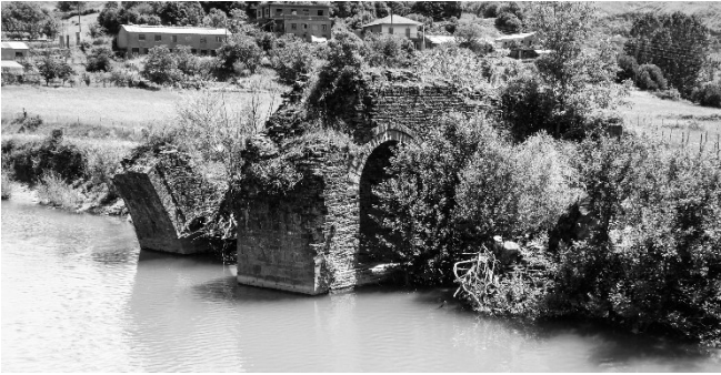
Fig. 1. Field research in the bridge of Kyra (photo of the authors).
