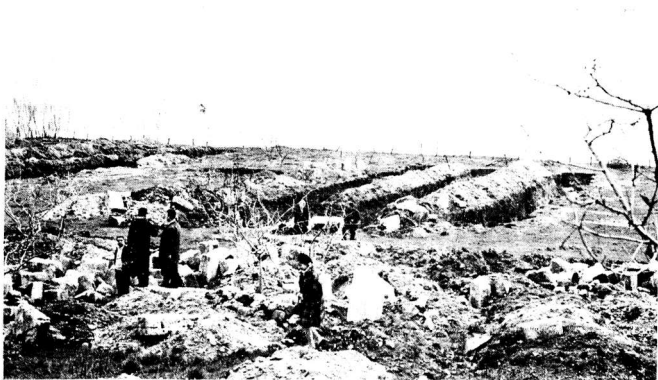
β. Ἀπὸ Δυσμῶν ἄποψη τῶν σορῶν ποὺ ἀπέθεσεν ὁ μηχανισὸς ἐξασφαλῆς (126)
