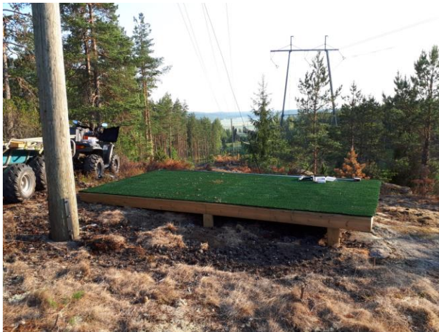
Figure 2: Disc golf platform built by the students
