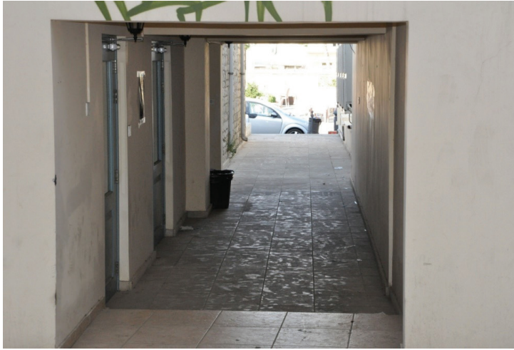
Figure 6: CUT Radio underpass
