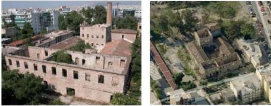
Fig. 5. Exterior views of the complex's current condition.
