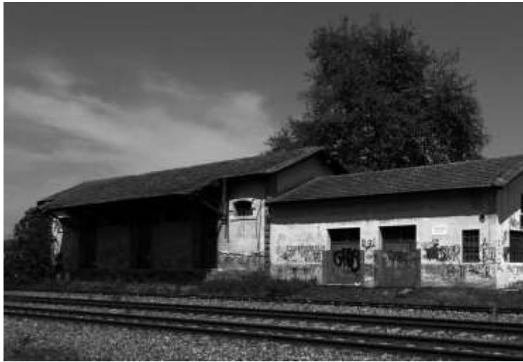
Fig. 11. Exterior view of the building's current condition [25].
