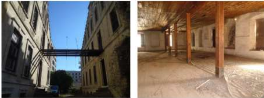
Fig. 8. Exterior and interior views of current condition.
