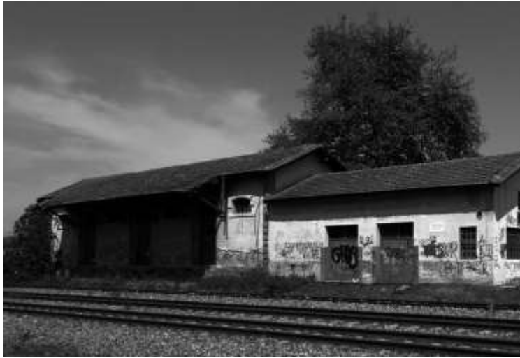
Fig. 11. Exterior view of the building's current condition [25].
