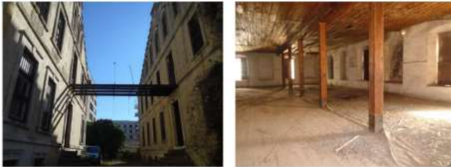
Fig. 8. Exterior and interior views of current condition.
