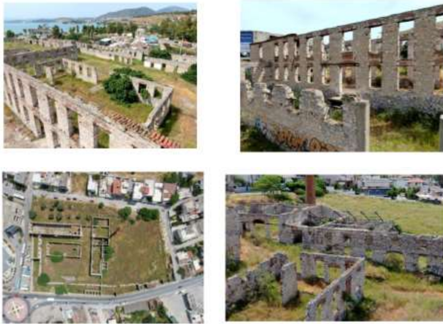
Fig. 2. Exterior views of the complex's current condition.
