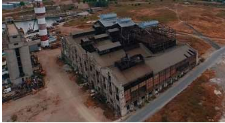
Fig. 14. Aerial view of the building's current condition [26].
