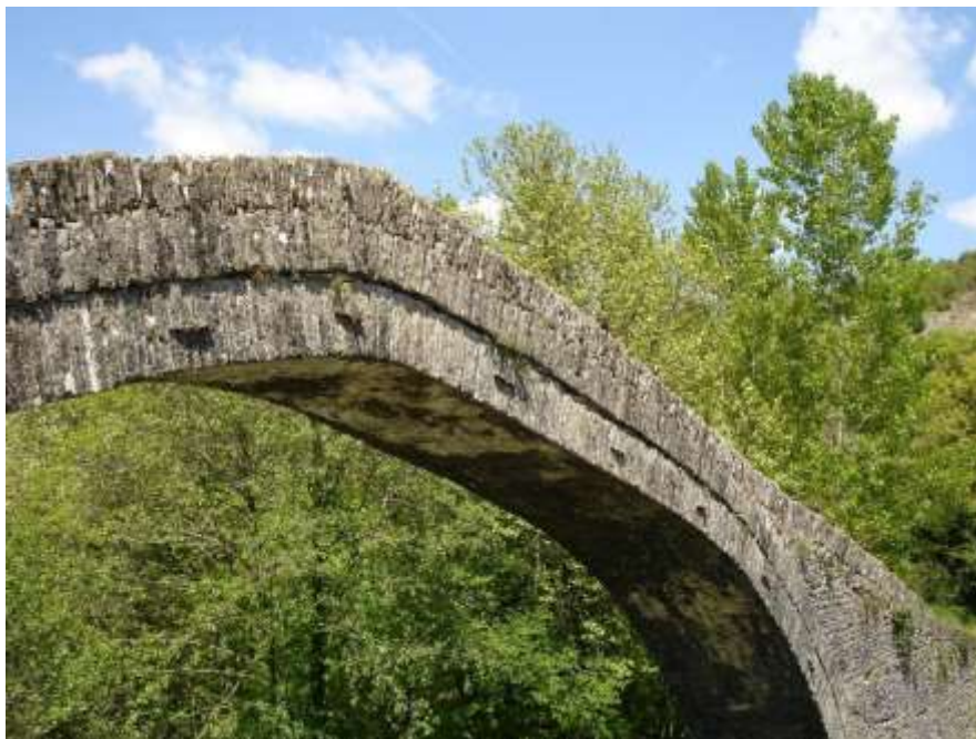
Fig. 3. The arch section tends towards its chord
