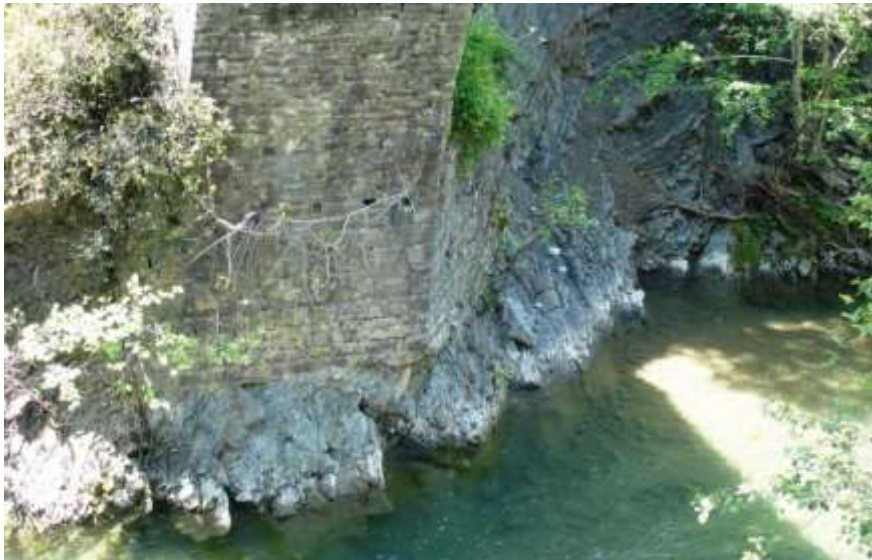
Fig. 5. Revelation of the foundation
