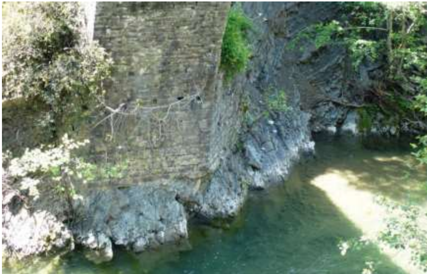
Fig. 5. Revelation of the foundation
